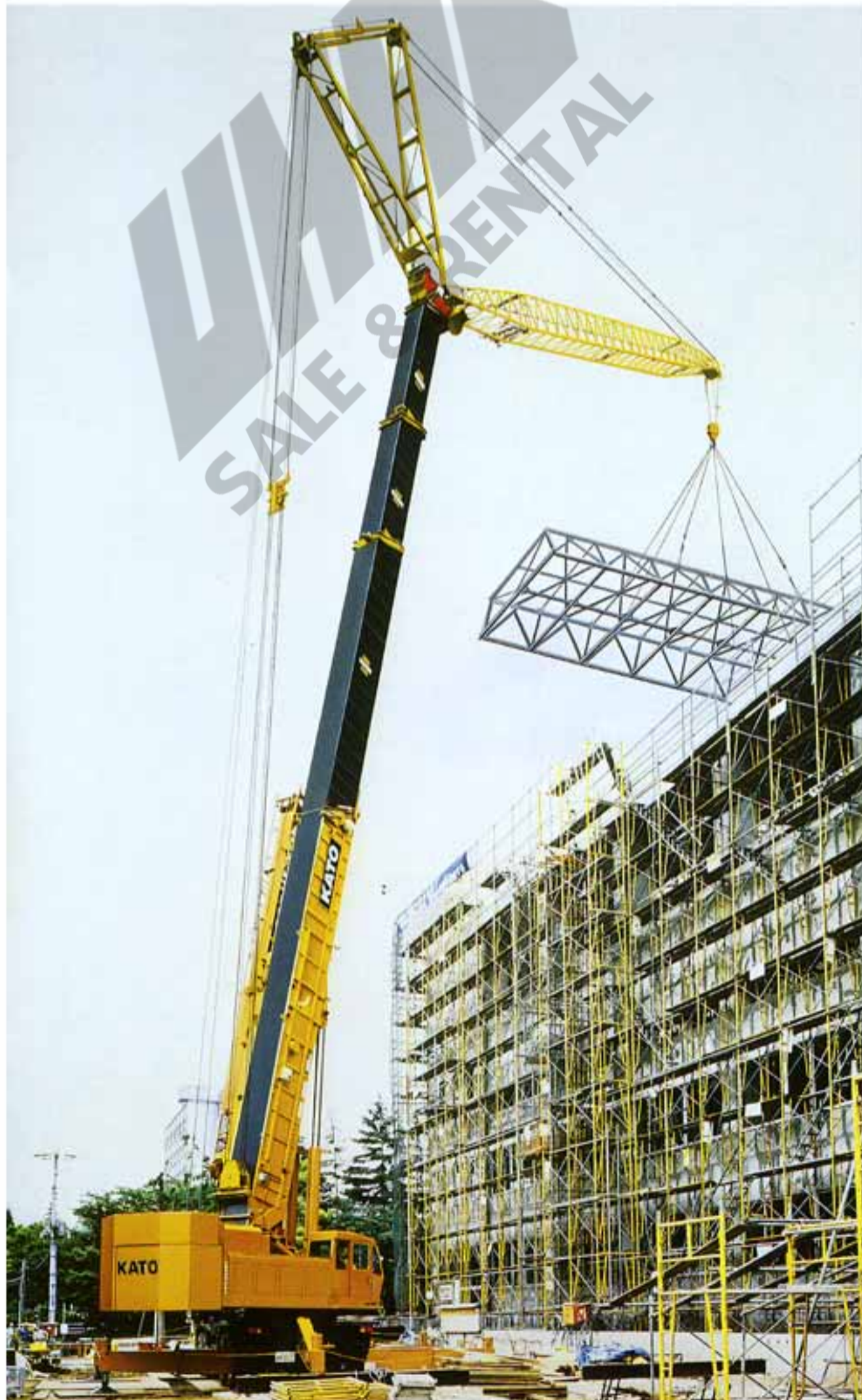
The installation of extra large load using the main boom and heavy lift jib. (Domestic model)
